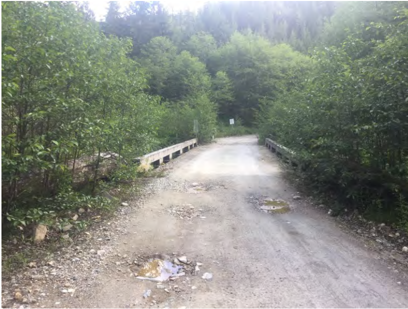
Approach from Right Bank when facing downstream
