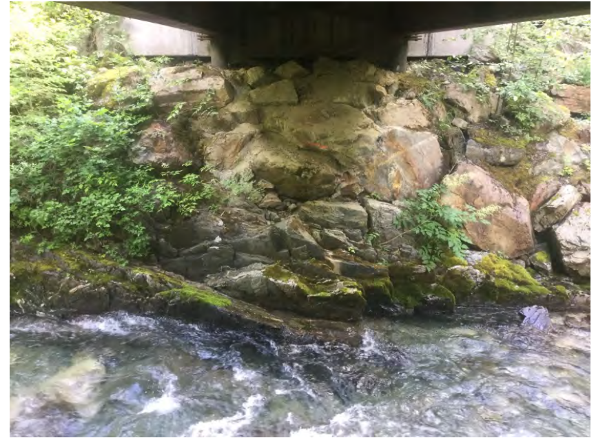
Left Bank Abutment when facing downstream
