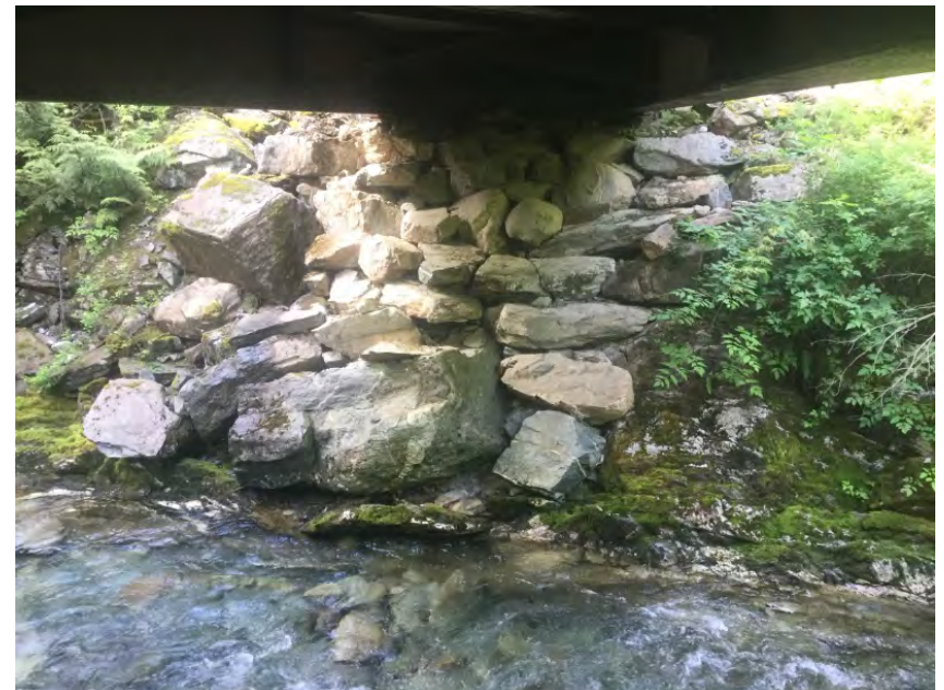
Right Bank Abutment when facing downstream
